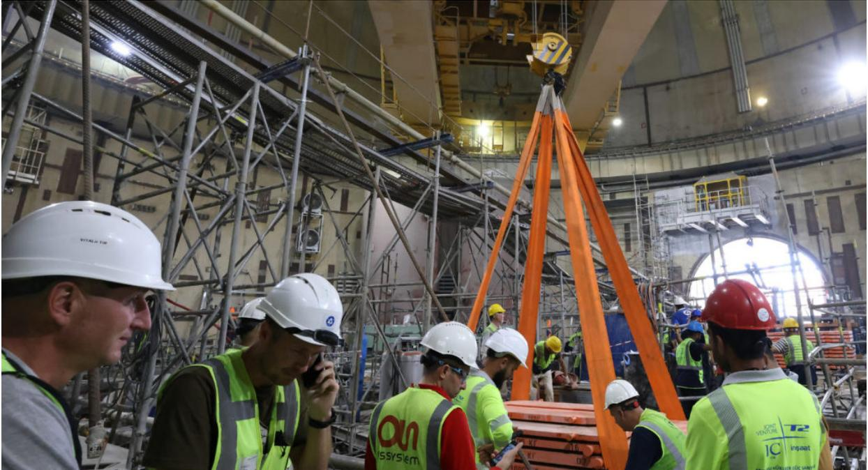
The polar crane, boasting a lifting capacity of 390 tonnes and a diameter spanning 41.5 meters, stands as a pivotal asset in the lifecycle of unit 1 at the new nuclear power plant. Initially tasked with lifting and maneuvering during the assembly of the nuclear reactor, it will continue to play a crucial role in subsequent years, facilitating the reloading and inspection of the reactor, as well as delivering nuclear fuel to the specialized reloading machine.
