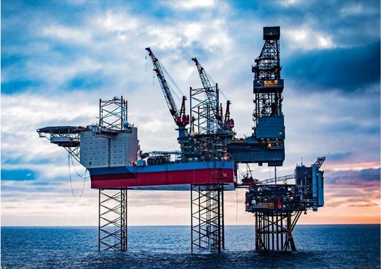
*Jackups of the CJ70 design, like the Noble Intrepid (pictured), typically have a higher variable deck load than semisubmersibles. However, the jackup's VDL may be negatively affected in some weather conditions if it's deployed close to the 150-m water depth boundary.*
